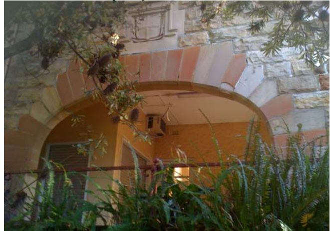
Detail of north-east stone verandah showing dressed stone arch and stone crest
