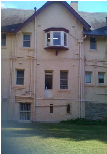
Part view of rear (east) elevation of Duntrim
