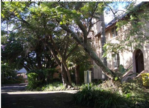
View of main façade and driveway approach, showing significant garden elements
