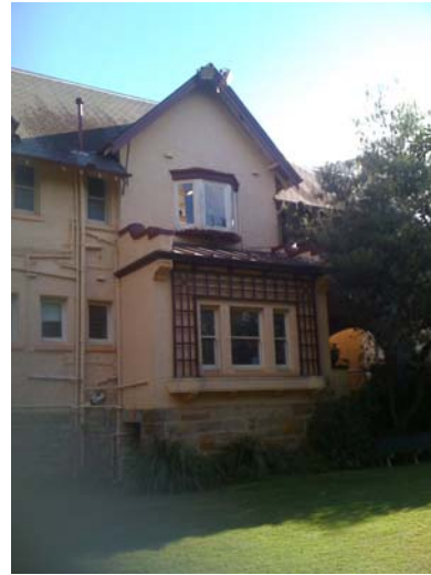
Part view of rear (east) elevation of Duntrim
