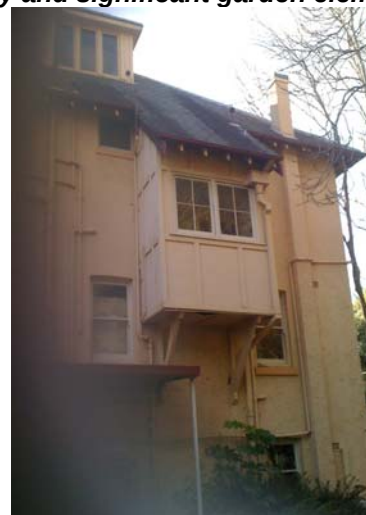
Part view of southern elevation of Duntrim
