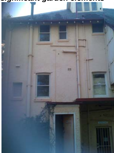
Part view of southern elevation of Duntrim
