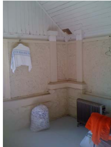
Interior details: view of enclosed balcony to upper level
